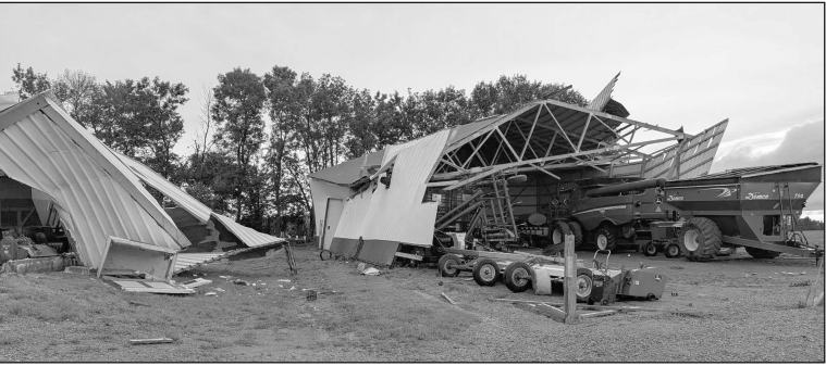
On Wednesday, a tornado touched down near Hartland and destroyed buildings on a nearby farm.
