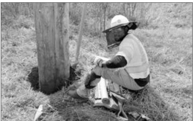
A crew foreman with Osmose Utilities Services carries out an inspection on a powerline pole along Hwy 13. About 13 crews of four people each have been working on similar inspections throughout the county for the past two weeks or so.
