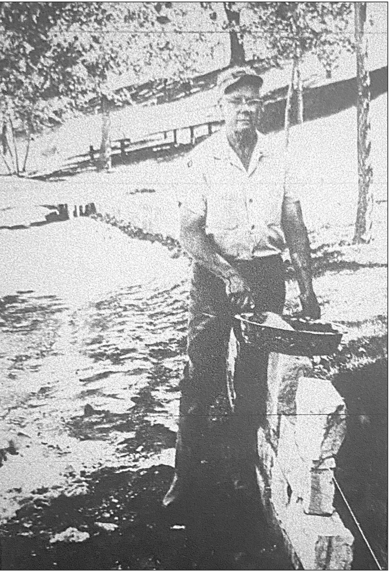
50 YEARS AGO - PLANNED RETIREMENT - Harold Mitchell was working on his retaining wall along Lake Elysian when the Argus photographer stopped by Monday. He retired as an instructor of the Mankato Area Vocational Technical Institute last month, but says he has at least three years' work on his home out on the lake. Retirement is something he and his wife have planned ever since they were married, Mitchell said.
