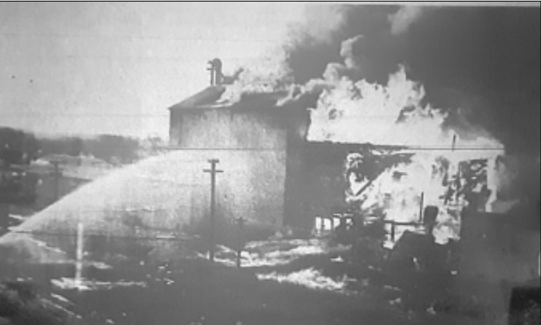
The GTA Elevator and Mill, which was built in Janesville in 1873, burned to the ground Tuesday, April 3, 1973.
