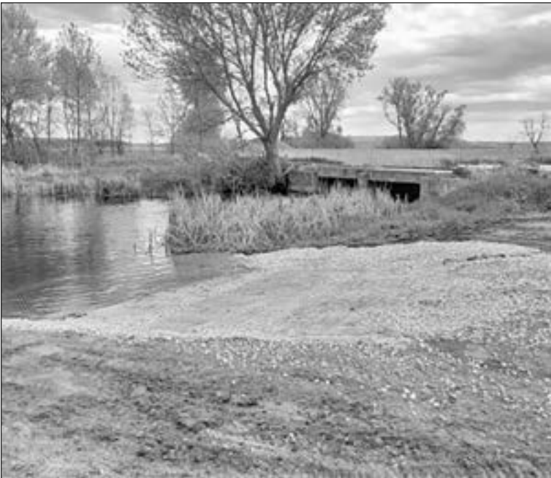
A new boat ramp was installed at Blowers Park in 2024, allowing access to Moonan Marsh and Watkins Lake.
