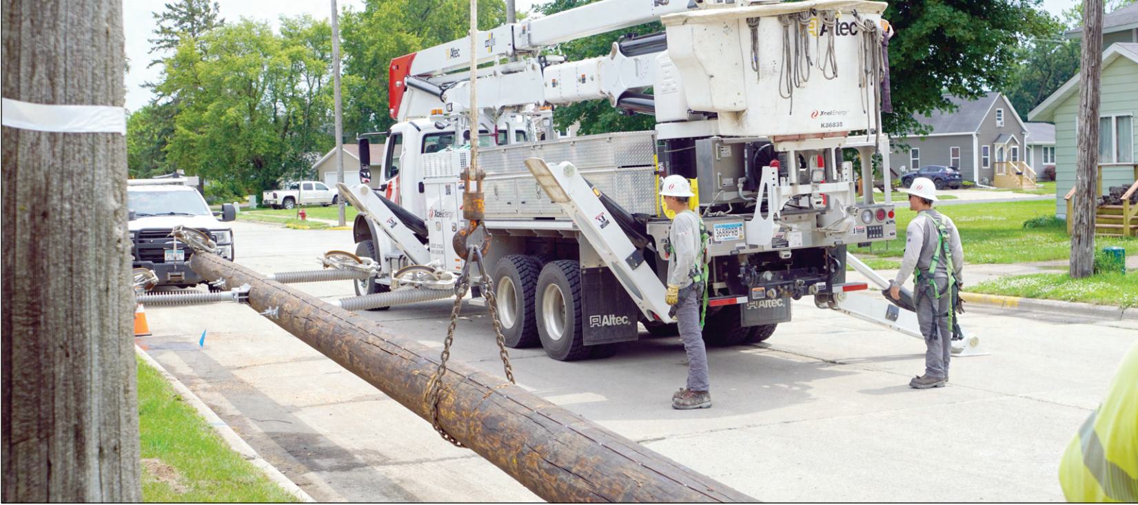
GETTING THE JOB DONE - Waseca local and Xcel Energy employee Bradyen Edwards, left, and fellow employee Cole Tallege were completing the final block of the Xcel Energy pole replacement project and service update along 4th Ave SW (next to old Bird’s Eye) on Wednesday, July 1, 2026.
