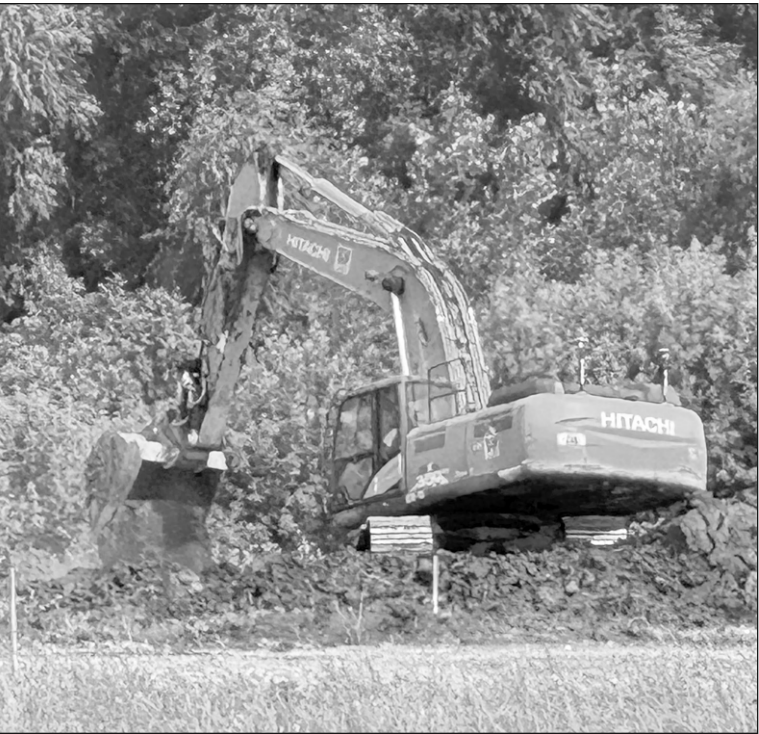
GRADING AND LEVELING -A lot of earth is being moved at the site of 17 lots in the City of Waseca's Clearwater Preserve subdivision. Some locations will be as much as five feet higher than they were before excavating began. Pioneer photo by Deb Bently
