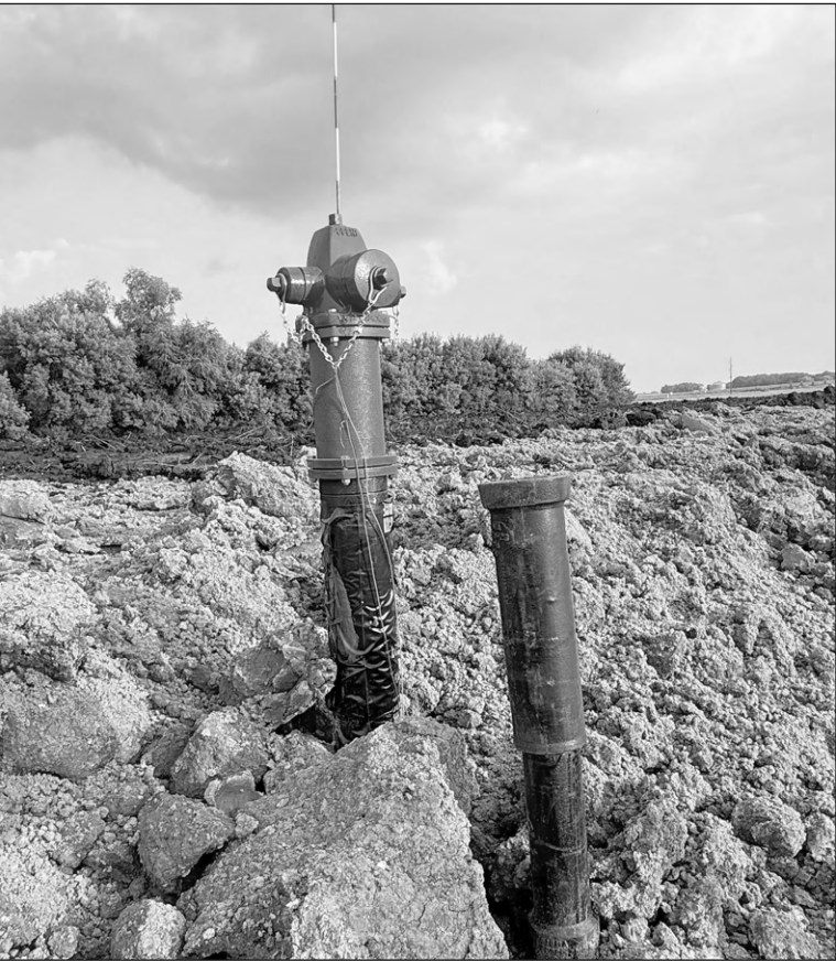
Water lines have been installed for phase 1 of the Clearwater Preserve subdivision at the southeast corner of Waseca. As this water hydrant shows, when sufficient earth and rock are brought in, some areas will be between three and five feet above their original level.
