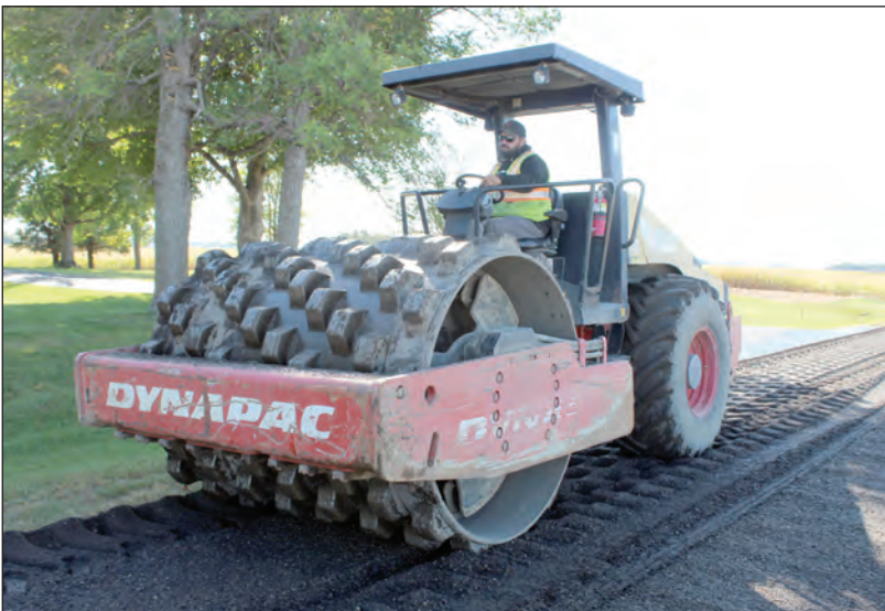
The “sheeps’ foot” compressor is the first machine to begin compacting the “reclaimed” asphalt after it has been lifted off of its former road bed. Pioneer photo by Deb Bently
