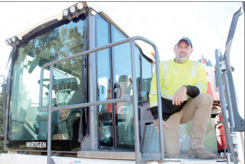
Ulland Brothers Inc. began the work of “rehabilitating” C.R. 64 bright and early the morning of Monday, Sept. 24. Pioneer photo by Deb Bently
